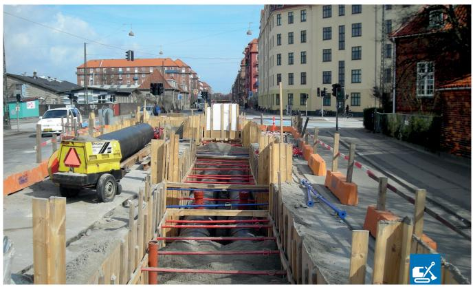
From March 2006 to March 2010, Aarsleff has carried out new district heating pipes and renewal of existing pipes in the centre of Copenhagen as well as in the districts of Vesterbro and Valby. The district heating system in Copenhagen consists partly of a concrete channel system with underground concrete structures and partly of pre-insulated copper and steel pipes. Heat is supplied by means of hot water and steam.
