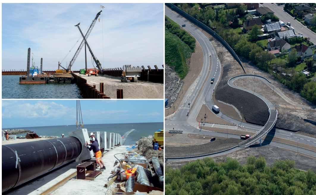
DN 1100 mm pipeline with ballast.
