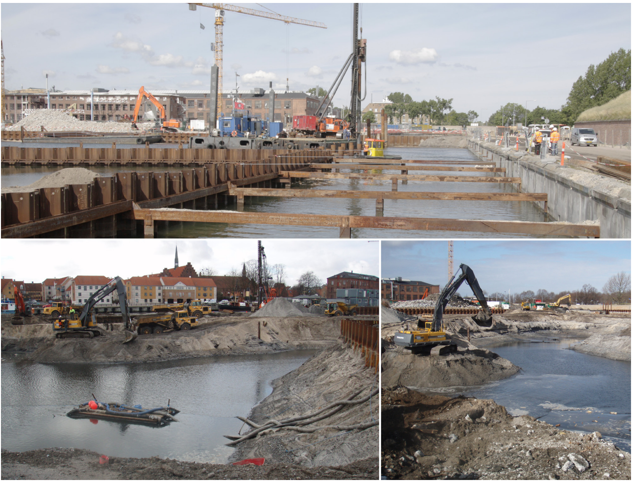
All sheet pile structures are permanent structures which will face the harbour basin or the moat when completed.
