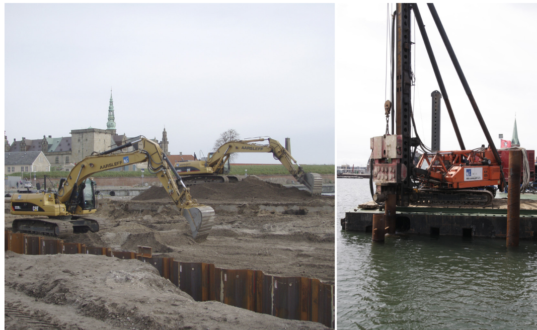
The soil work is another story. 140,000 cubic metres of soil is not a gigantic amount, but when clean earth and contaminated soil are mixed and have to be handled in different ways, excavating the soil must be planned carefully.
