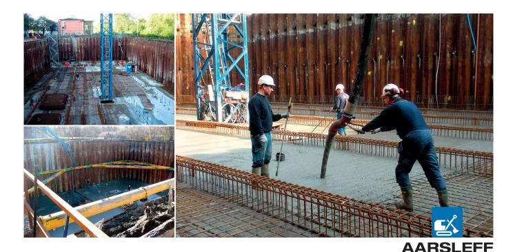
In the period between 2008 and 2011, Aarsleff constructed an equalisation basin in Aarhus with a capacity of approx. 16,000 cubic metres. The basin was constructed as a square-shaped structure, and Aarsleff's work comprised concrete work and sheet piling, installation of anchors, excavation and installation of precast concrete units.
