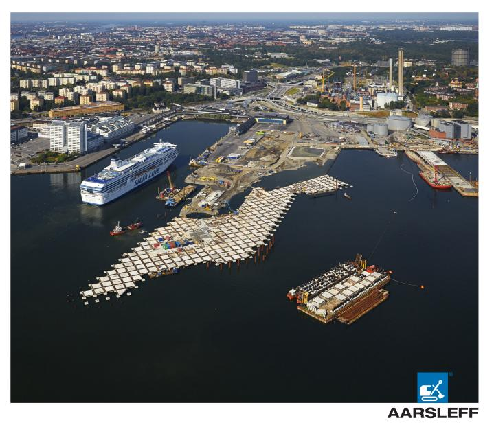
In a design and build contract, Per Aarsleff A/S has extended the largest of Stockholm's harbours, Värtahamnen by 85,000 square metres. The work was carried out from 2013 to 2016. The existing harbour areas were transformed into a new urban area.
